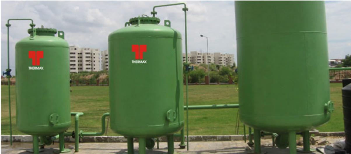
Thermax offers a wide range of filtration systems standardised on the basis of specific velocities for each type of filter. Filters are available with single 5-way valve operation & multiple valve operation depending on the flow rate & the application. Filters are available in MS (painted), FRP & HDPE construction.
